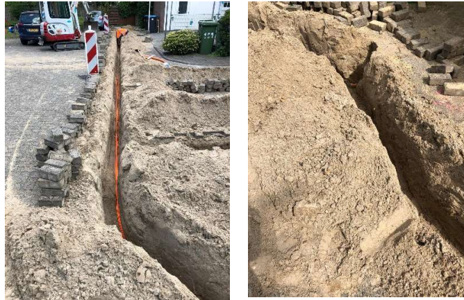
Figures 4 and 5. Laying of cable
