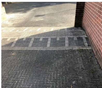
Figure 13. Example of a proper speed bump
