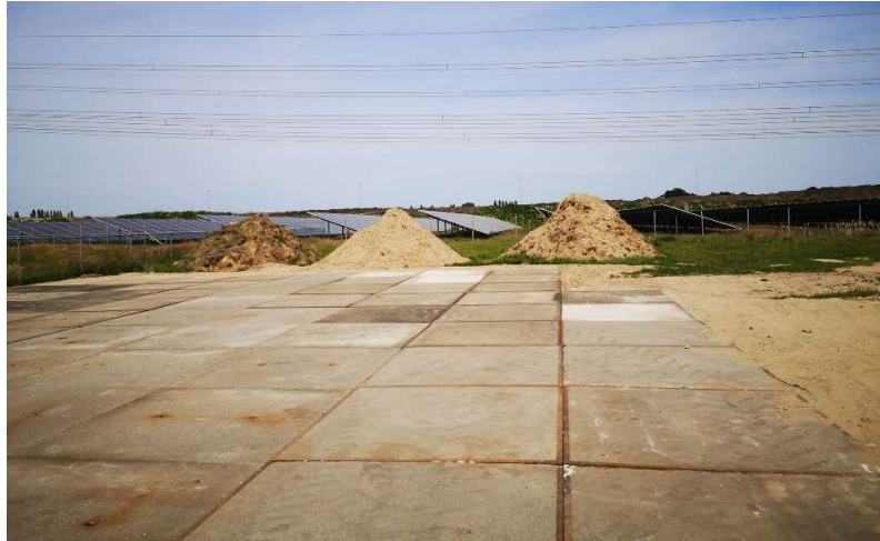
Figure 8. Soil stored at the soil bank.
