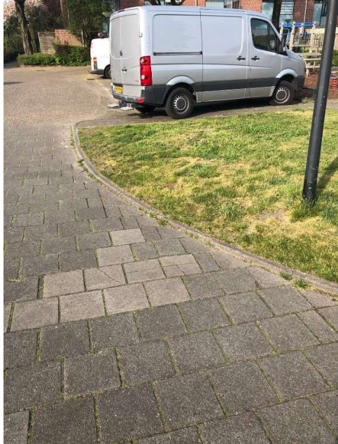
Figures 4 and 5. Places where a tree has been cut down. This tree continued to cause extra work every few years after which they decided to cut it down. You can still see this in the newer tiles with which they replaced the old ones.
