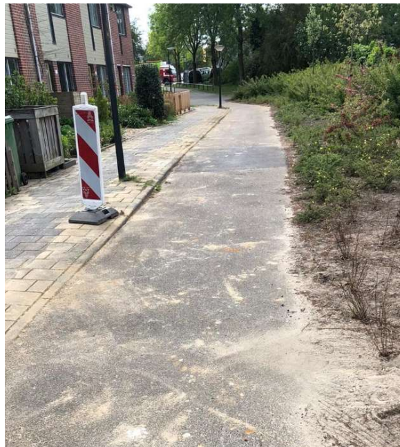
Figure 3. The asphalt part in Griffiersveld
