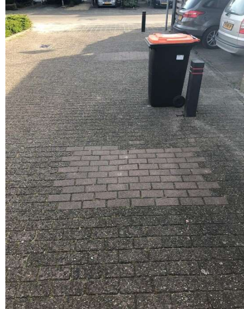
Figures 4 and 5. Places where a tree has been cut down. This tree continued to cause extra work every few years after which they decided to cut it down. You can still see this in the newer tiles with which they replaced the old ones.
