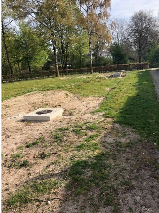
Figures 10, 11 and 12. Water sewerage in the Griffiersveld area. All the rainwater is lead to a canal nearby.
