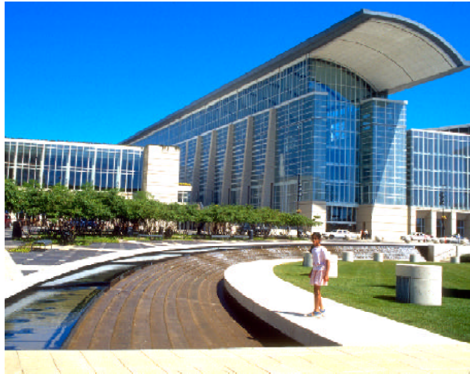
Figure 2.24 The recent expansion of McCormick Place has doubled the number of events, which attract more than 3 million people annually.
