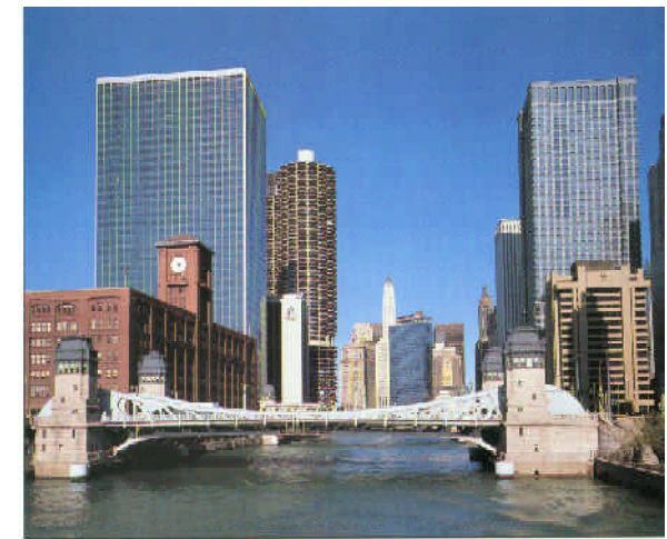
Figures 2.9 and 2.10 Bascule bridges, like Chicago's architectural landmarks, are part of its unparalleled design heritage and legacy of engineering innovation.
