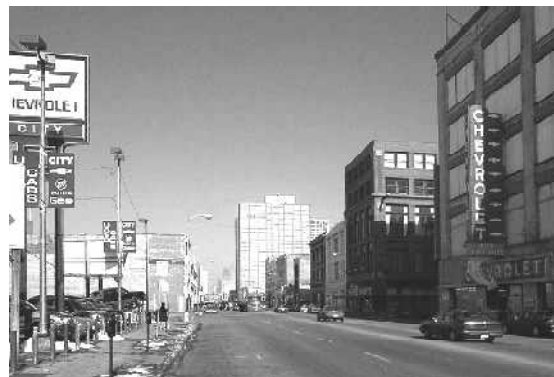
Figure 5.18 The South Michigan-Wabash-State Corridor today.
